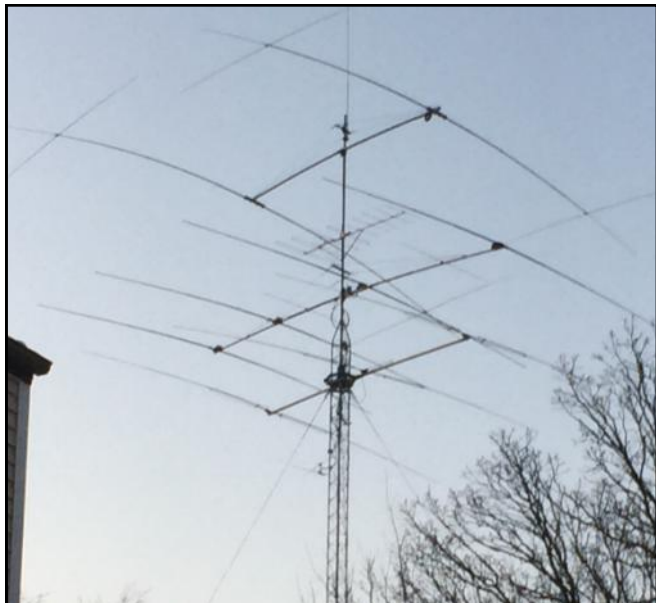
WØAD's antenna stack on 80' of Rohn 45G
